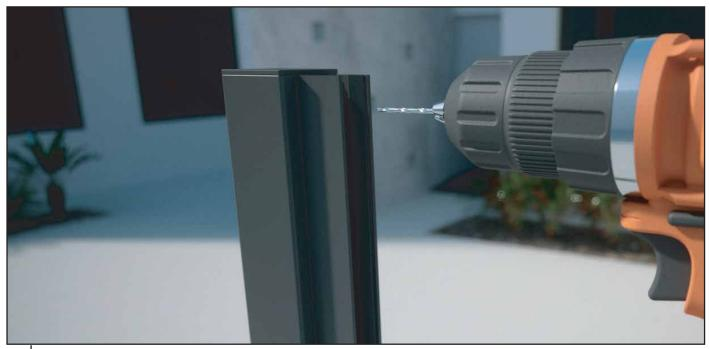
9 To allow for the top end plate, position the side frames 1/8inch less than the desired height and drill pilot holes in side frame for mounting. Attach side frame to post or mounting substrate using appropriate fixings (fixings not supplied). Repeat for all side frame locations.
