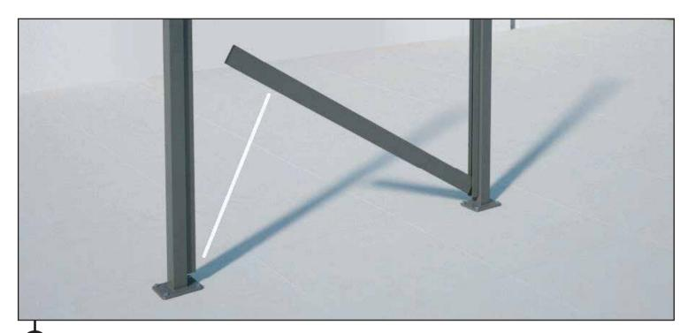
10 Install first slat into side frames directly onto bottom plate (no spacer required). Lever slat in at an angle. Ensure the first slat is level. Patented aluminum side frame legs will hold slats firmly in place.
